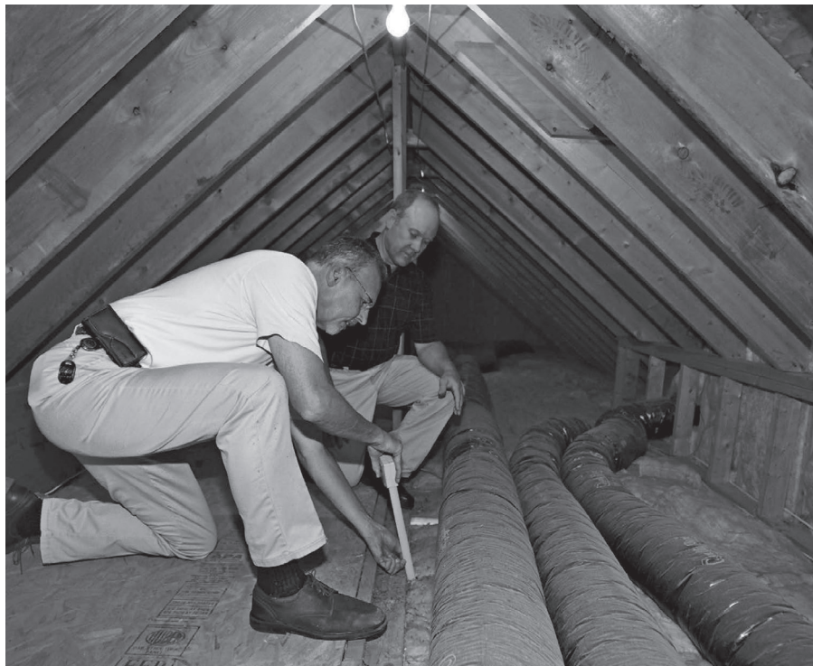
photo courtesy of the Piedmont Electric Membership Corporation
