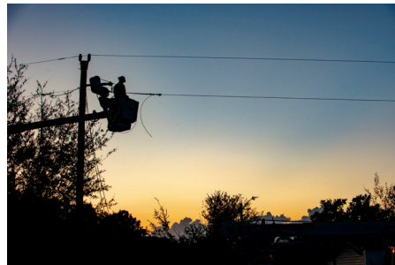
Keeping buildings, trees and other obstructions out of the right-of-way gives our linemen room to work.
